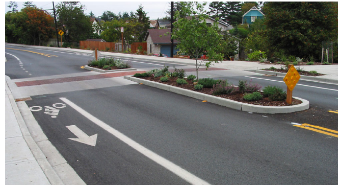
Crosswalks with refuge islands reduce crossing distances for pedestrians on wide streets. Source: Ramsey, County, Future Road Project.
