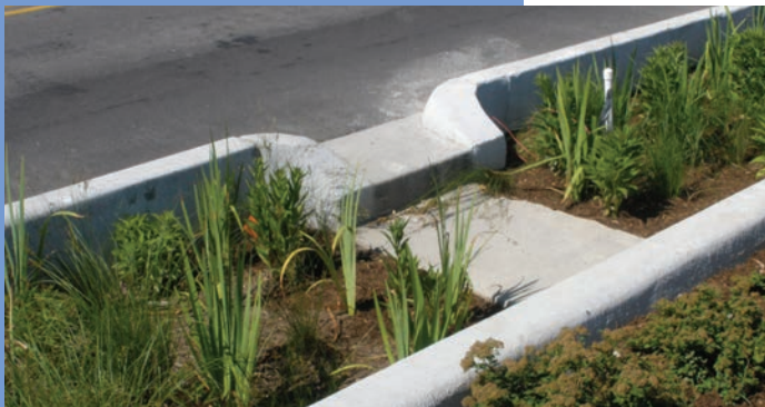
Example of bioswales treat runoff
